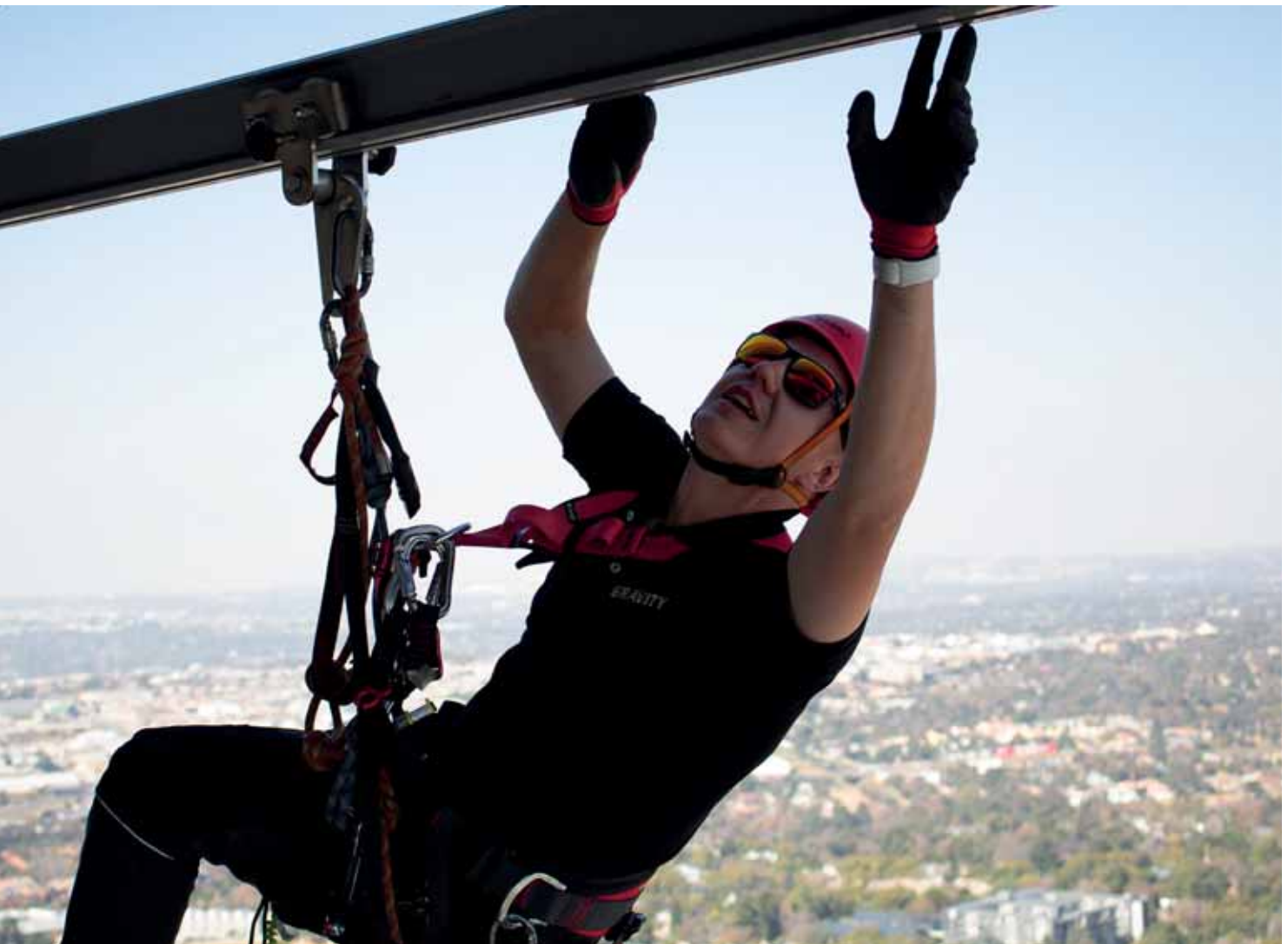
Martyn Cilliers doing maintenance operations on the Leonardo building, using C.A.M.P. gear and the Gravity Securail. Martyn Cilliers realiza el mantenimiento del edificio Leonardo, utilizando equipos C.A.M.P. combinados con Gravity Securail. Sandton, Johannesburg, South Africa (courtesy of Gravity Gear Pty Ltd, ph. Ethan de Witt).
