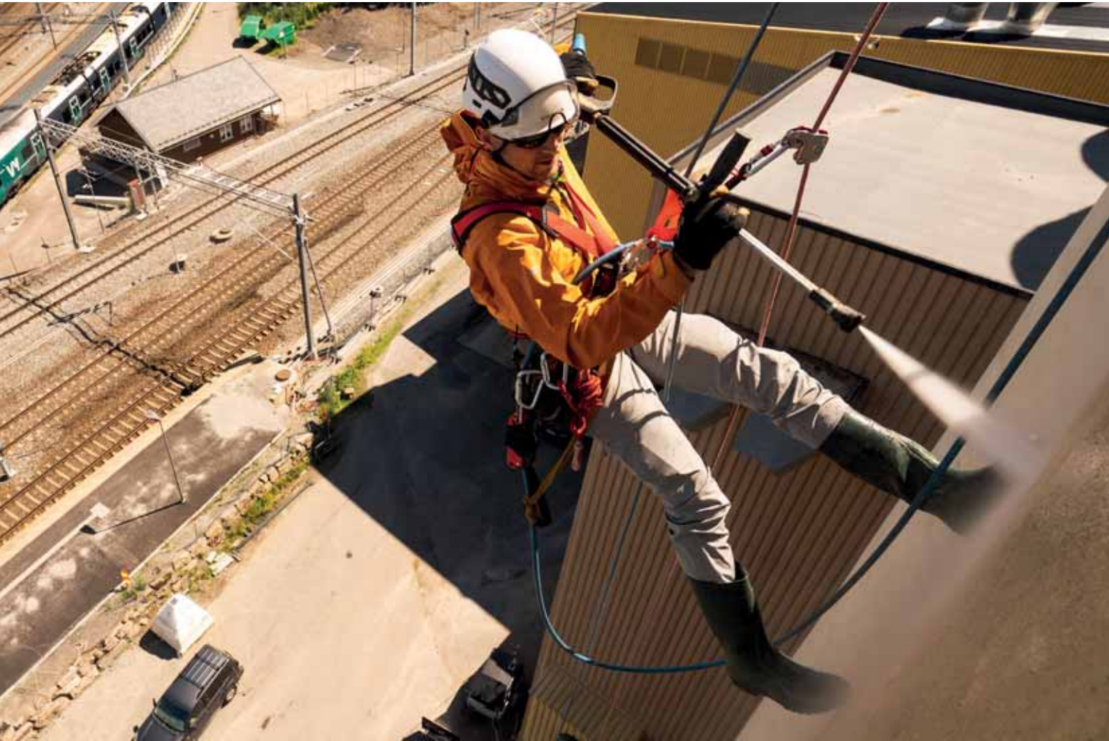
Torbjørn Solheim carrying out high pressure cleaning operations on the Felleskjøpet building. Torbjørn Solheim realiza tareas de lavado a alta presión en el edificio de Felleskjøpet. Eidsvoll, Norway (courtesy of Varri AS, ph.Kyrre Buxrud).
