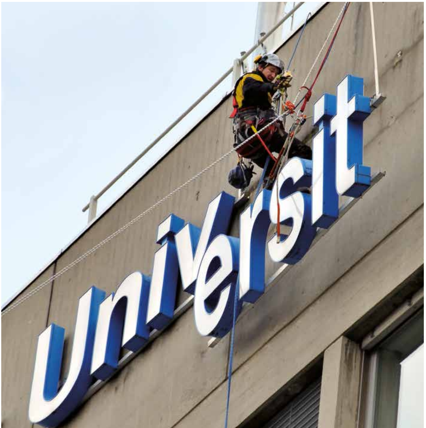
Dismantling of a neon sign at the University Hospital of Geneva. Desmantelamiento de un rótulo luminoso en el Hospital Universitario de Ginebra. Geneva, Switzerland (courtesy of Corde-Access SA, © Corde-Access SA).
